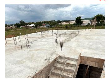
for about a month. Then supports will be removed and work will start on installing the electrical conduit in the walls. The walls are concrete blocks so workers will chisel out channels for the conduit and install it before the masons plaster the walls and cover up the conduit. Electrical, water and sewer conduits were installed in the roof and floor
